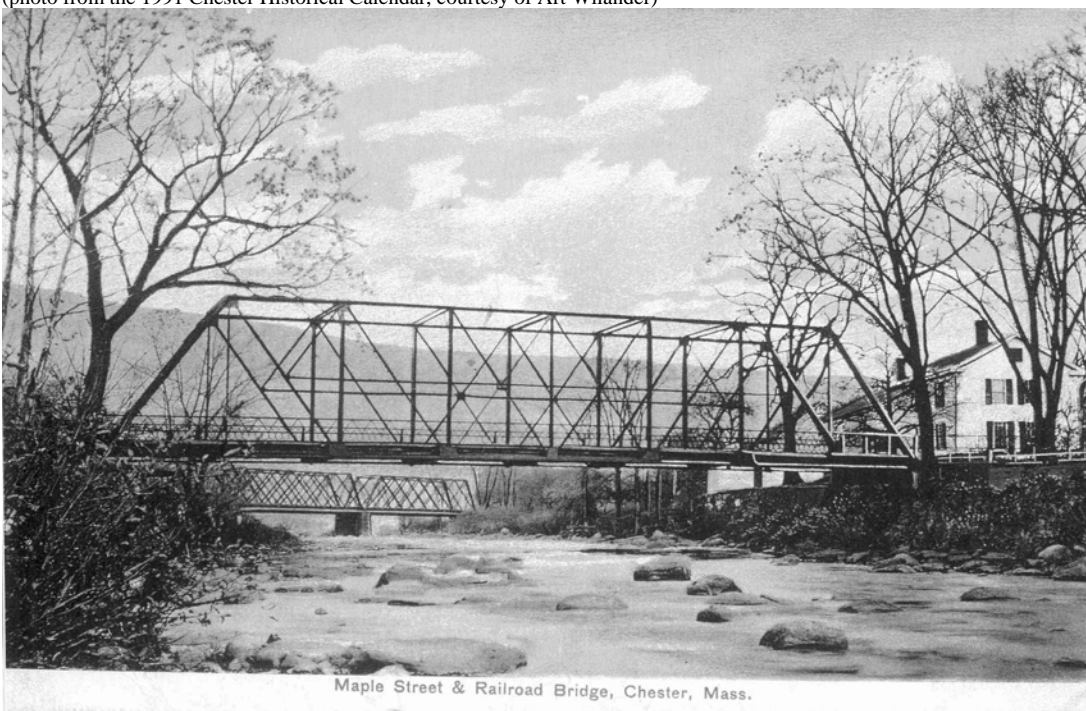
The “Pratt Through Truss” Maple Street Bridge circa 1910
